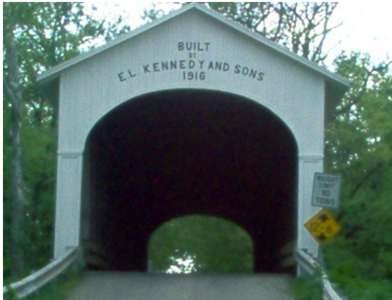
The Norris Ford Bridge
